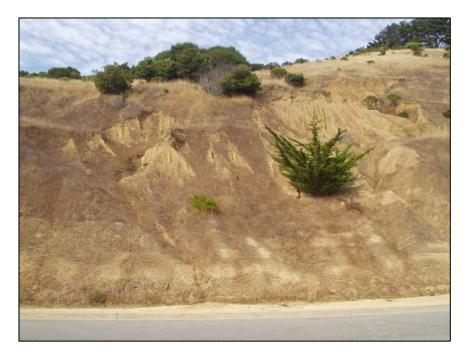
The following photograph illustrates the potential problem of providing a safe overland release of runoff. Site design should be conservative to help prevent a repeat of this situation, where runoff eroded its own path to the street below, completely bypassing the designed drainage facility:
